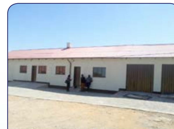
Homes of Safety and shelter at Khorixas after renovation (February 2014)
