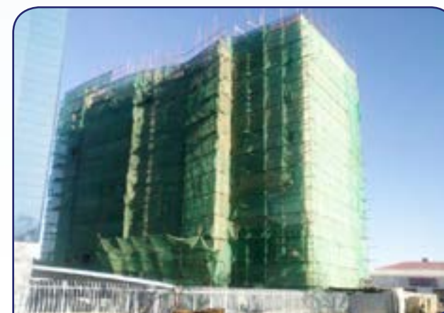
Ministerial Headquarter Juvenis, under renovation
