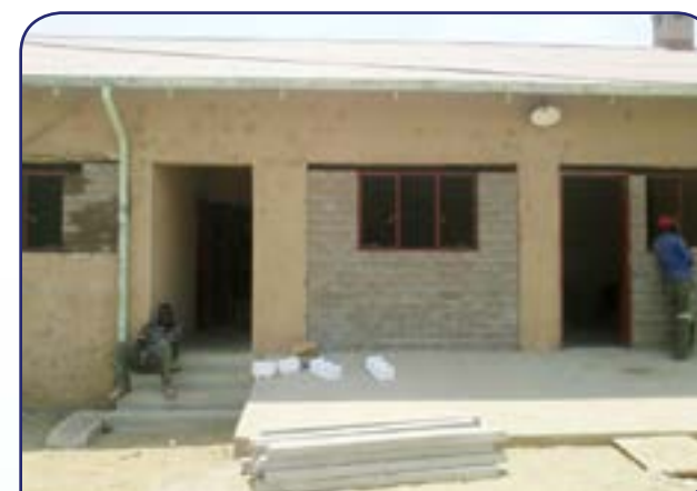
Above is a picture of the Home of Safety under renovation in Khorixas (2013)
