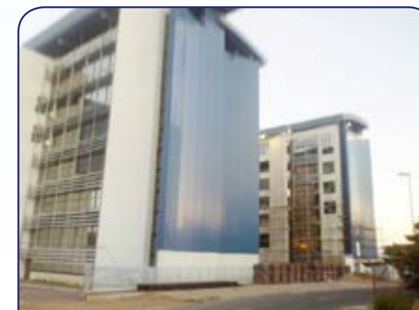
The Ministerial Headquarter Juvenis Building after renovation (March 2014)
