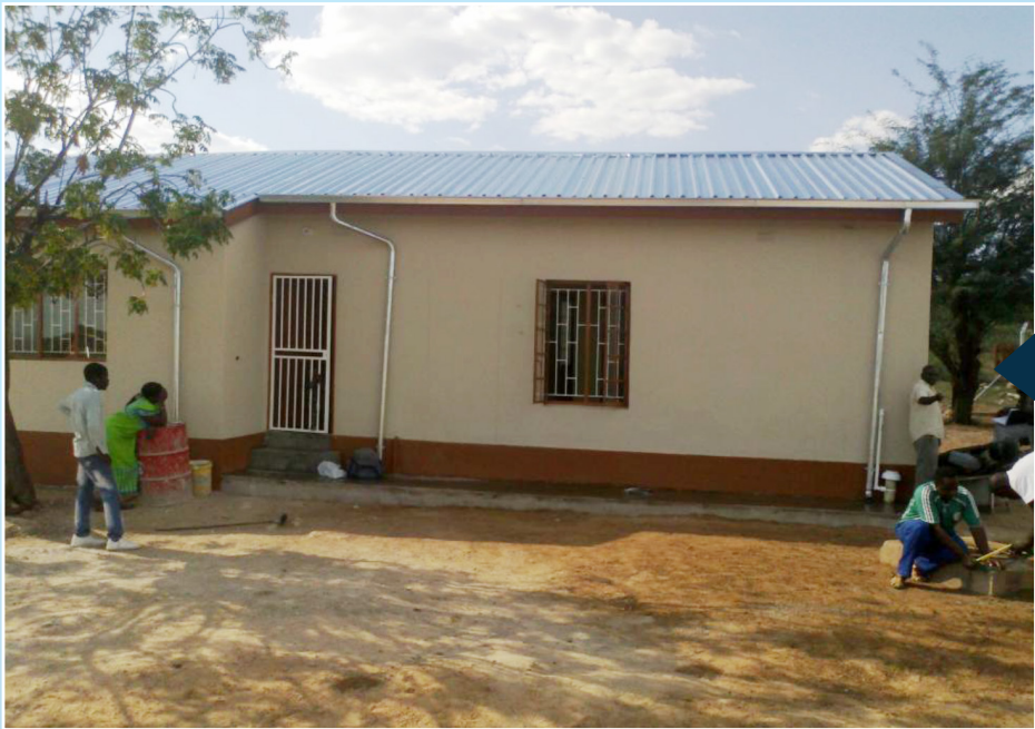
A building in Epukiro, Omaheke region, converted into an office after renovation.
