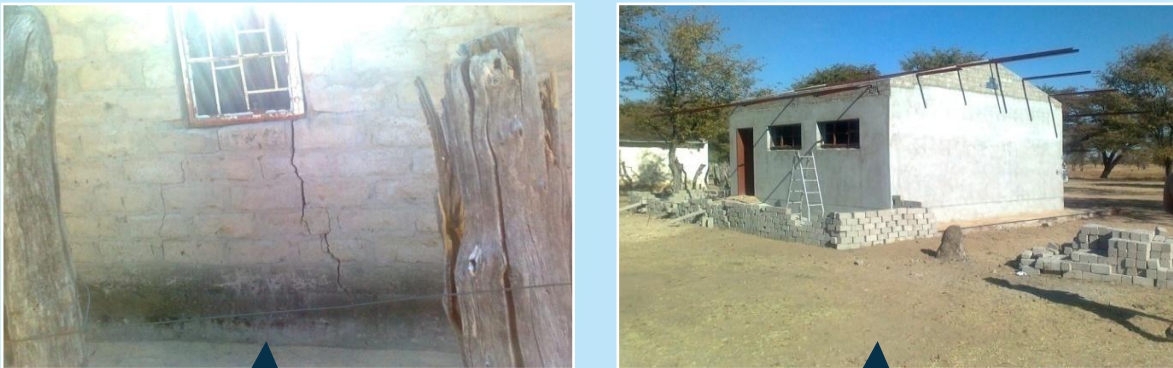
Oshikulufitu dilapidated ECD Center under reconstruction in Oshikulufitu village – Anamulenge Constituency
