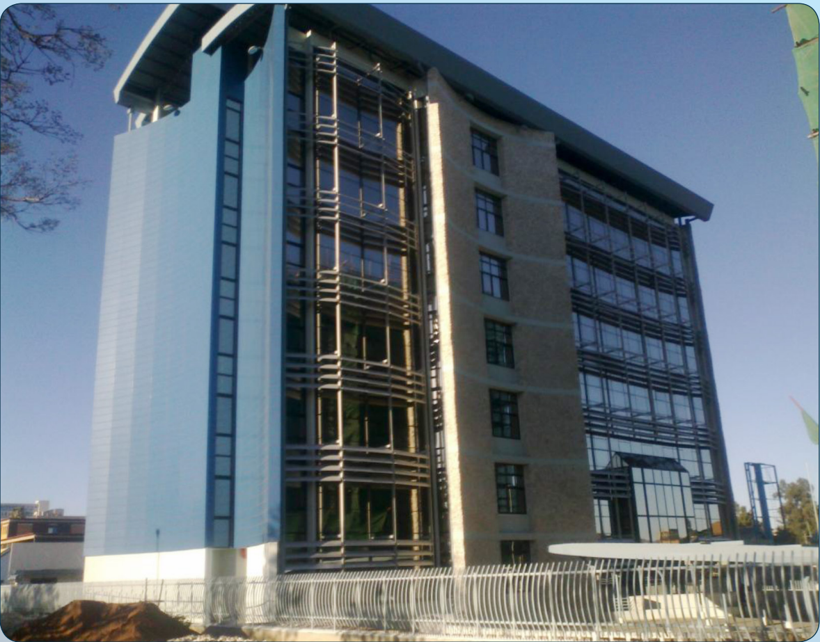
Newly constructed Ministerial Head Office in Windhoek
