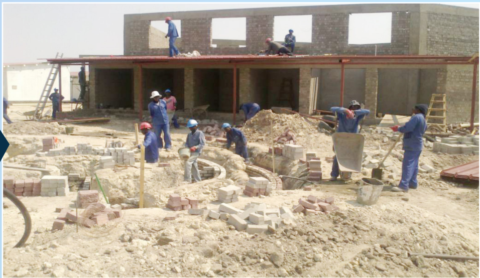
Outapi Craft Centre under construction
