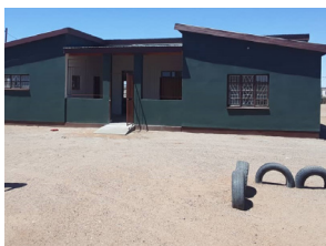
Renovation of a Standard ECD Centre, Berseba Constituency, Bethanie.
