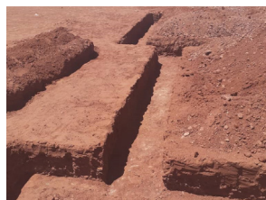
Foundation trenches for the construction of a Standard ECD Centre in Keetmanshoop Rural, Aroab.
