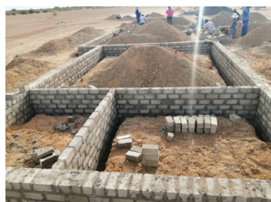
Construction of an Standard ECD Centre in Karasburg East, Wortel
