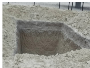
A dry pit toilet under construction at the nahas ecd centre, omuthiya constituency
