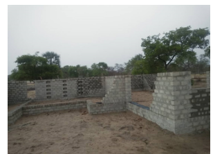
Construction of a Standard ECD Centre in Okankolo ECD centre, Onekotale village, Okankolo Constituency, Oshikoto Region.
